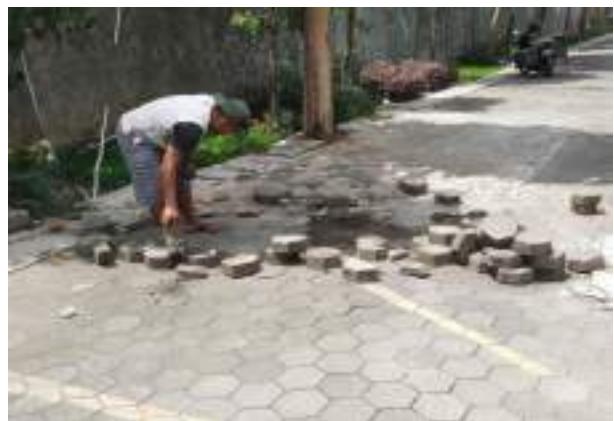
Proses perapian paving block
