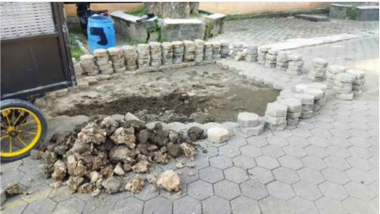
Proses perbaikan paving blok timur Plaza Umar Kayam
