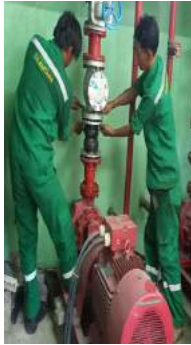
Penggantian Flexible Joint Main Pump Hydrant & Diesel Hydrant
