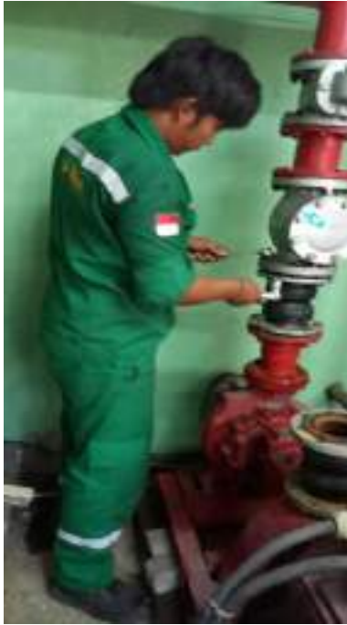
Penggantian Flexible Joint Main Pump Hydrant & Diesel Hydrant
