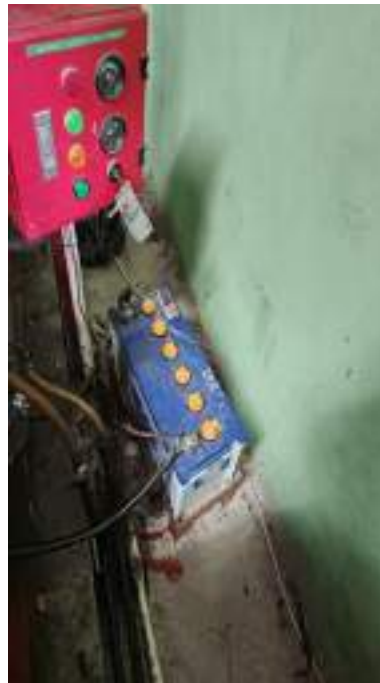
Perbaiki Panel Auto Start Diesel Pump & Ganti Accu Diesel Hydrant
