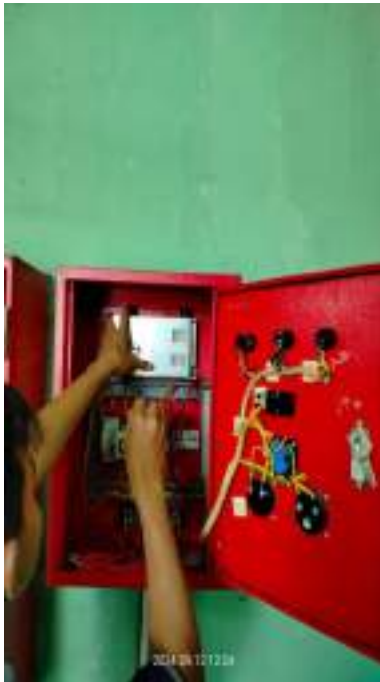
Penggantian Auto Charger Accu Diesel Hydrant dan Service Diesel Hydrant
