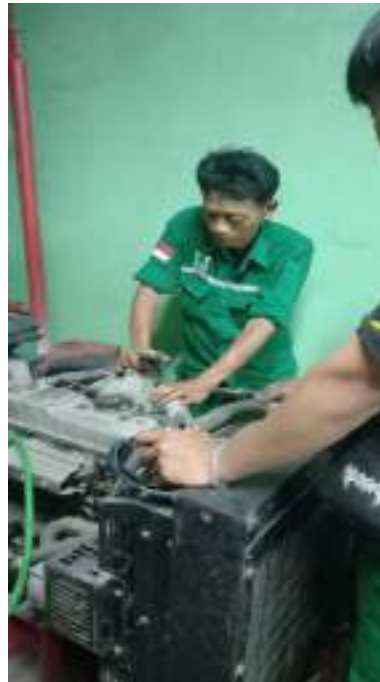
Penggantian Auto Charger Accu Diesel Hydrant dan Service Diesel Hydrant
