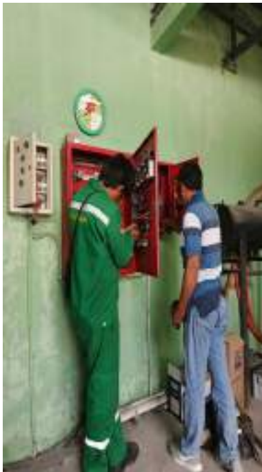
Perbaiki Panel Auto Start Diesel Pump & Ganti Accu Diesel Hydrant
